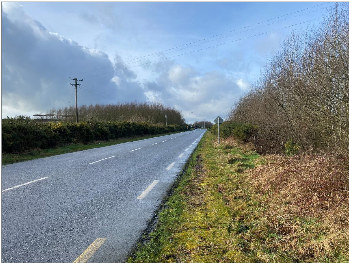
Plate 4-18: Example of a section of the existing Tinnycross Road in which part of the underground electrical cabling route is to be located, categorised as Buildings and artificial surfaces (BL3), with associate road verge, scrub and hedgerow.
