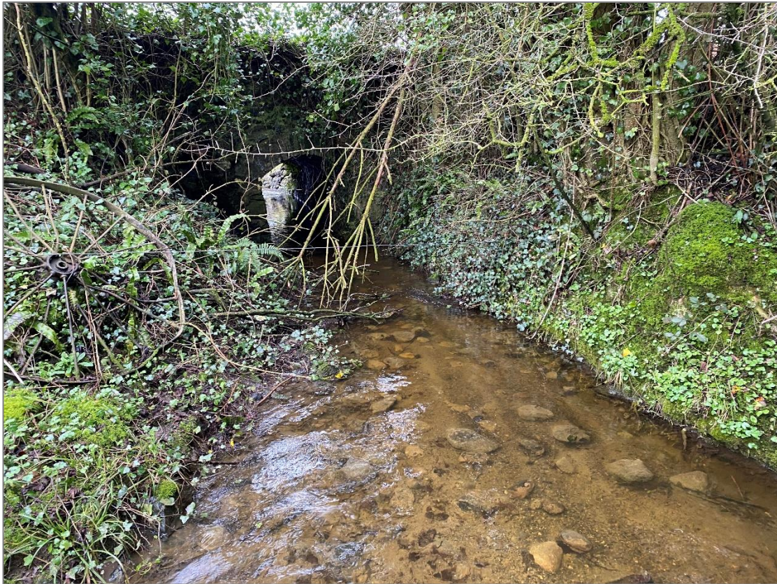
Plate 4-19: Example photo of an existing watercourse crossing occurring on the underground electrical cabling route (Watercourse ref. WC6).
