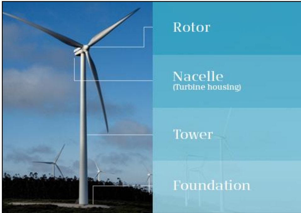
Plate 3-1 Wind turbine components
