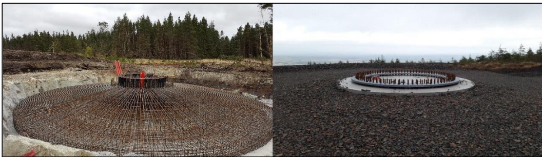
Plate 3-2: Turbine 'Anchor Cage' and finished turbine base
