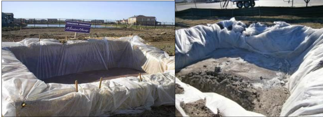
Plate 3-3: Concrete washout area
