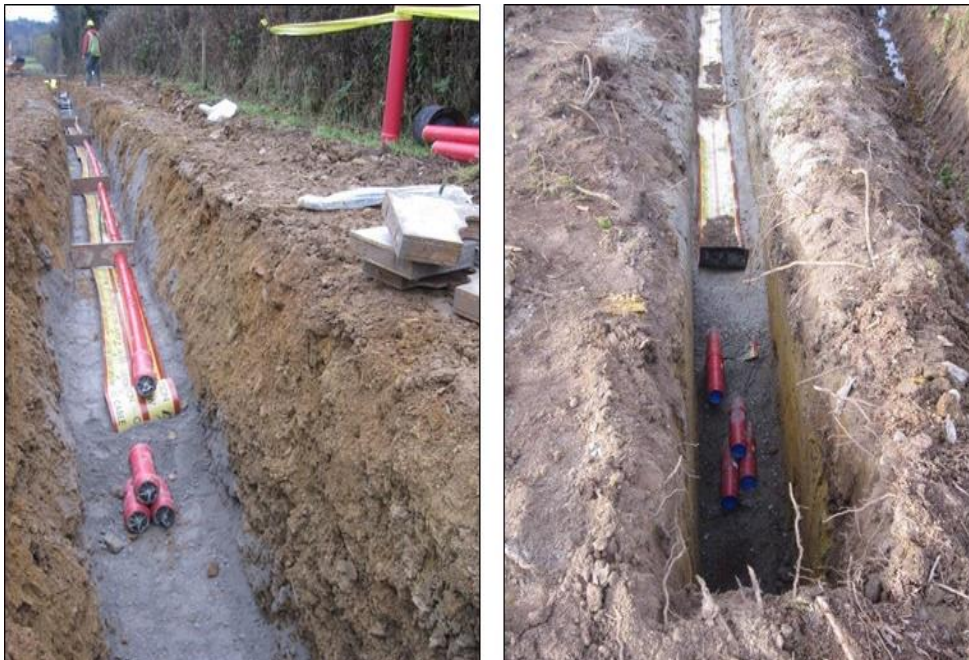
Plate 3-4: Typical Cable Trench View
